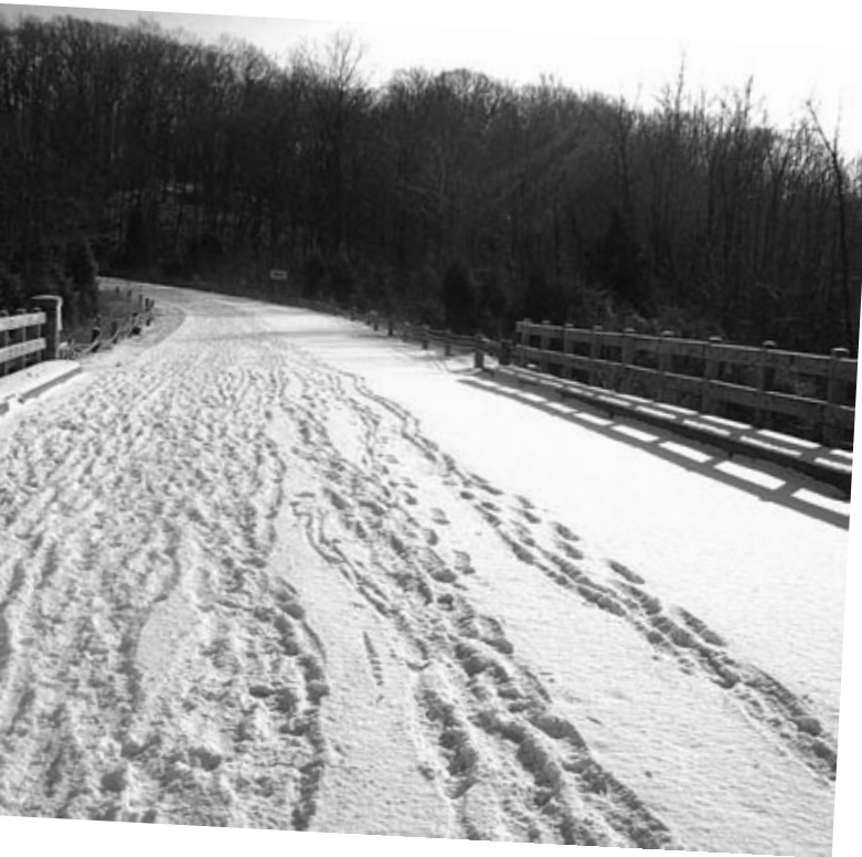
Hueston Woods Loop Rd. bridge over Four Mile Creek below the dam. The road was closed due to ice beneath the snow and all you can see are the hiker's footprints.
