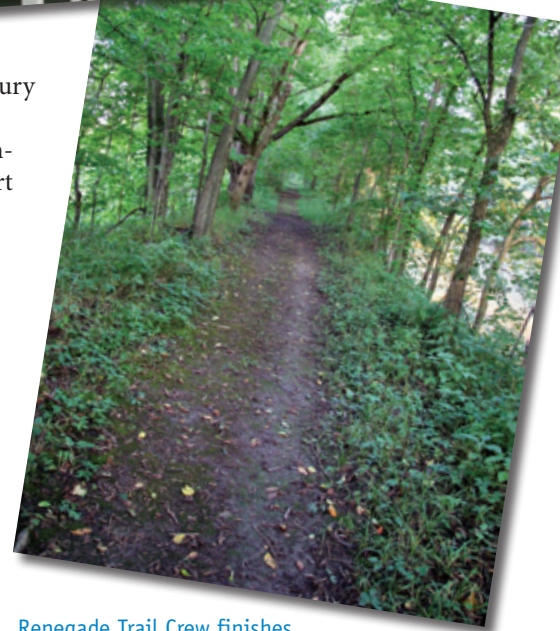
Renegade Trail Crew finishes the trail tread and a footbridge during a Buckeye Trail Crew Work Party near Napoleon on the Miami & Erie Canal towpath.
