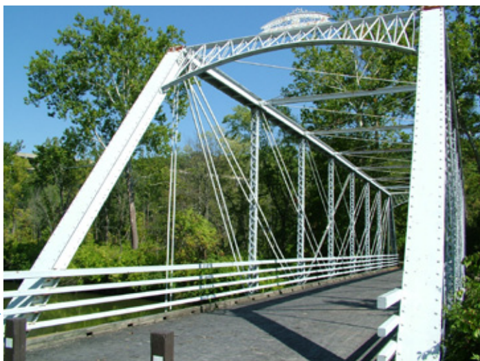
Station Road Bridge in the Bedford section. At the request of the National Park Service, the Buckeye Trail is not blazed on the canal towpath, so watch for directions on signs! . . . and always carry a map
