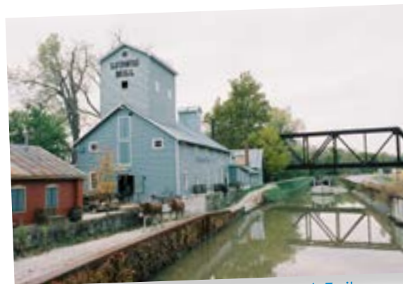
Ludwig Mill and canal boat, Towpath Trail in Providence Metropark
