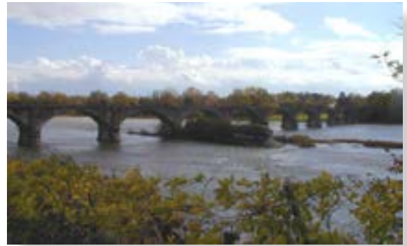
Old rail bridge over the Maumee River near Roche de Bout, Toledo's Farnworth Metropark
