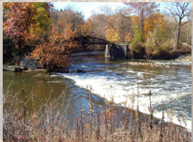
Bridge over the Cuyahoga River
