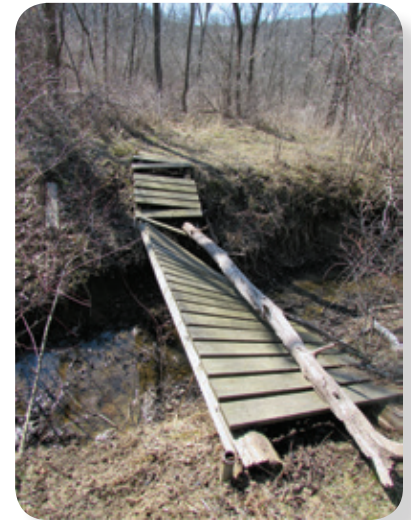
The condition of the previous bridge
