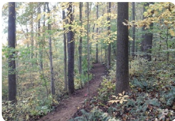
Newly finished trail at Bowerston
