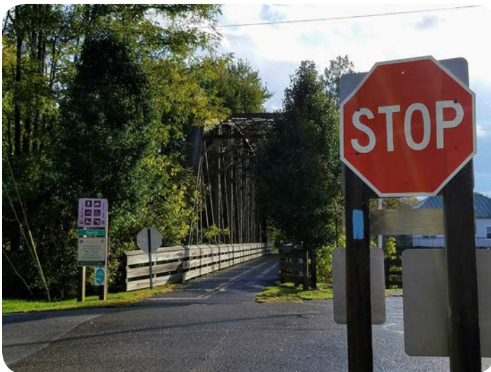
Morrow Old Rail Bridge
