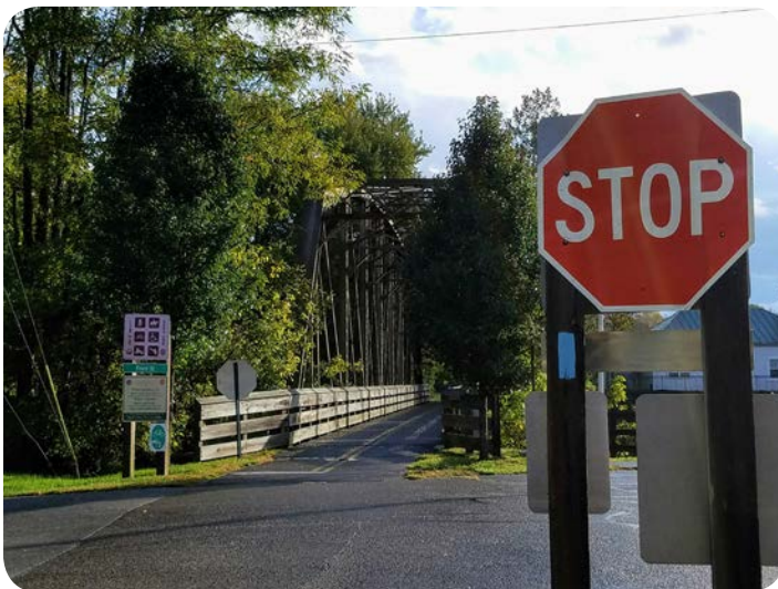
Morrow Old Rail Bridge
