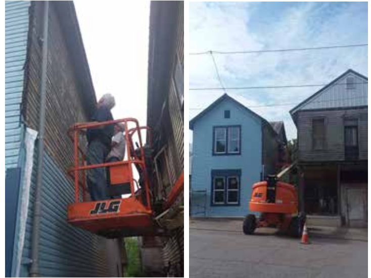
Steve & Herb working on 129. Photo by Richard Lutz
