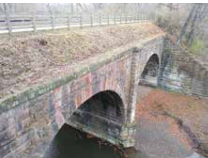
Old RR Bridge (pictured left).
