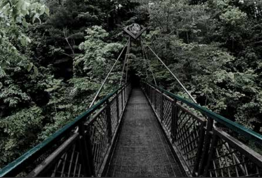
The A-frame Bridge by Cedar Falls.
