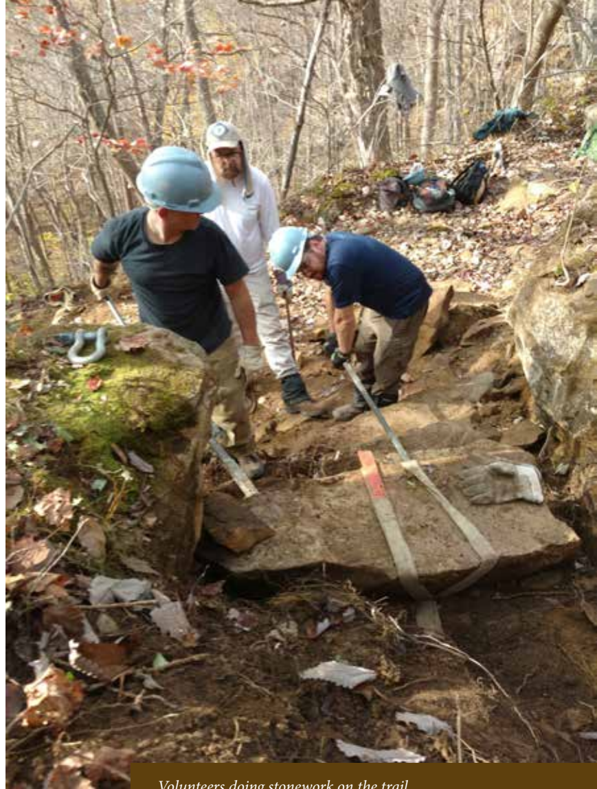
Volunteers doing stonework on the trail.
